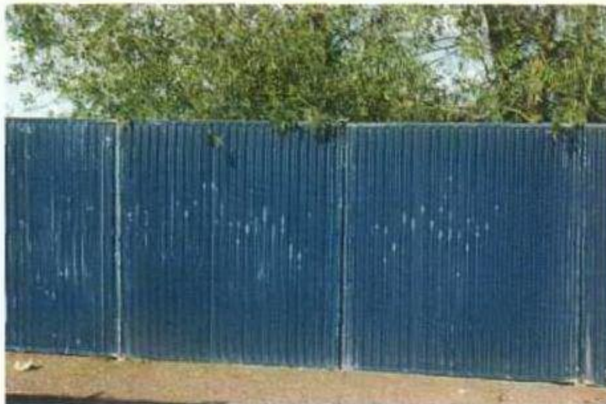
Figure 1 Typical Panelised Hoarding, to be painted offsite prior to erection.
