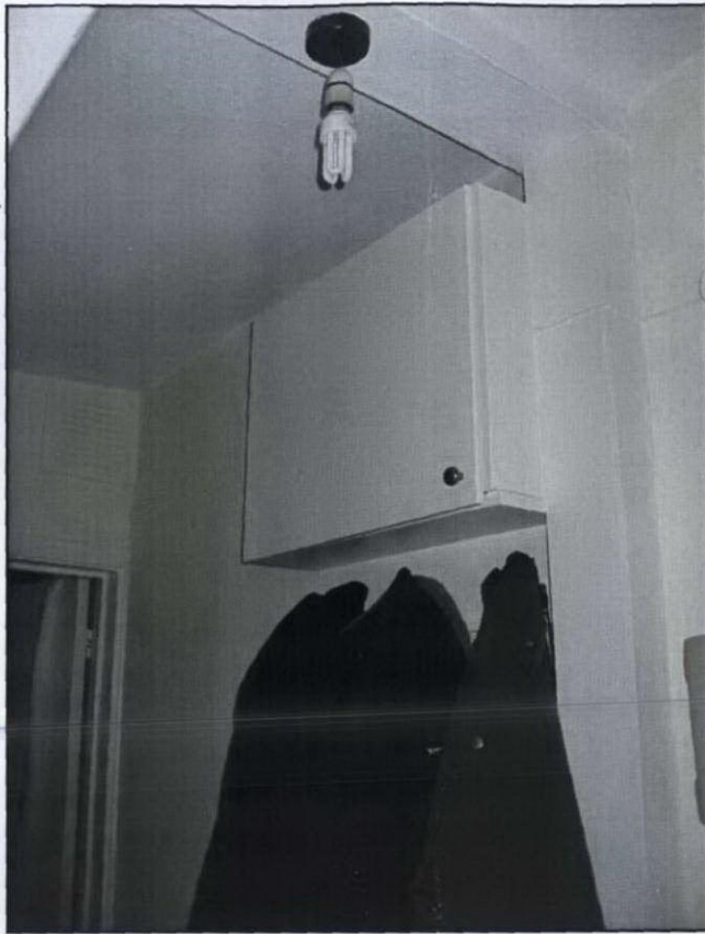
08 EXISTING CORRIDOR FINISHING
