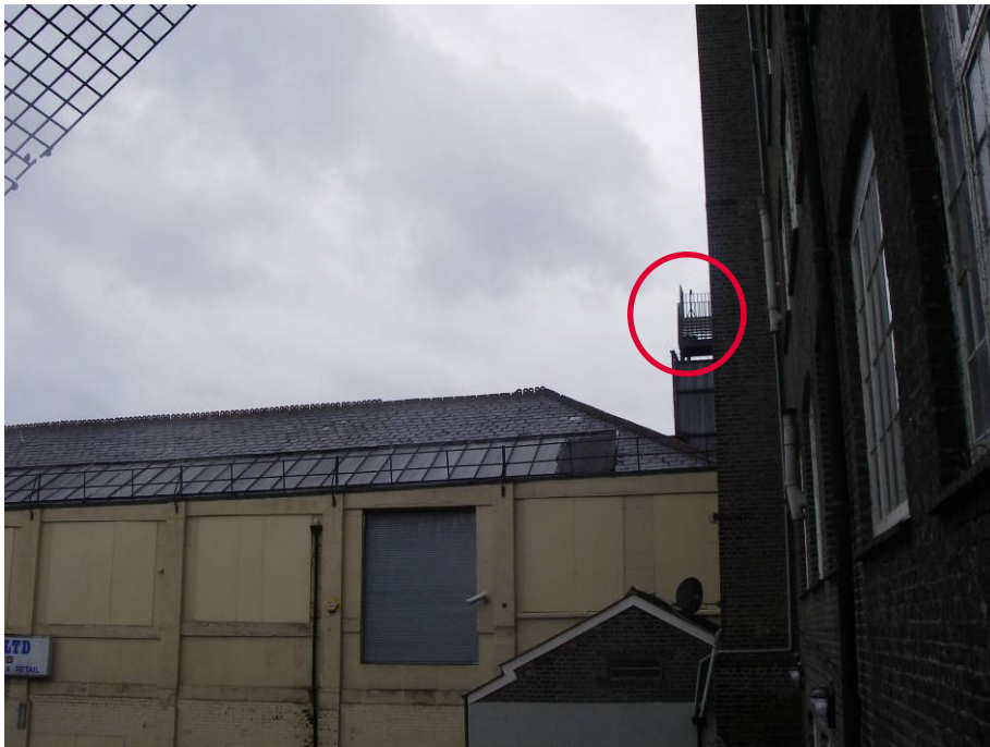
Figure C3: View South Towards Location N3 (circled)
