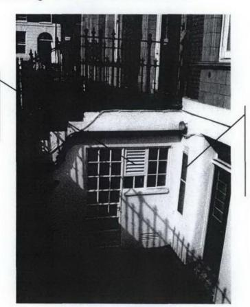
Proposed top glazing to be removed and timber Louver installed.
