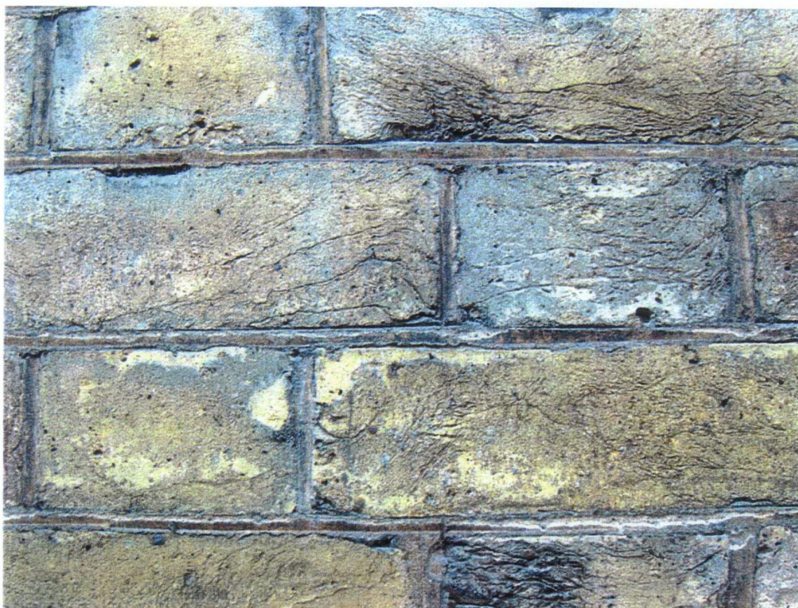
Photograph of an uncleaned area of the West elevation showing original pointing and brickwork
