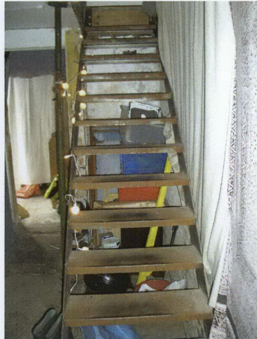
Existing steel staircase from Ground Floor Across prop supporting floor joists
