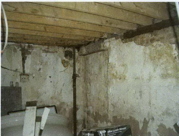
Rear Room, rear projection, showing new floor joists
