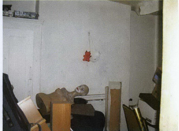
Rear Room chimney breast and party wall
