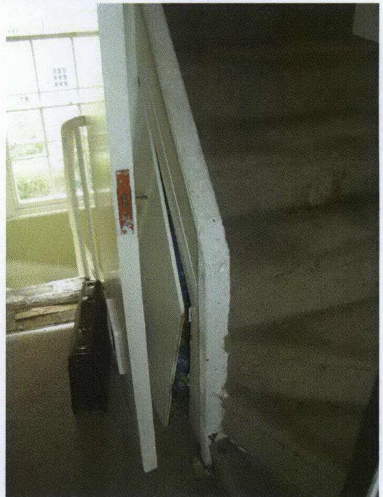
ACCESS FIRE DOOR AND STAIRS TO THIRD FLOOR
