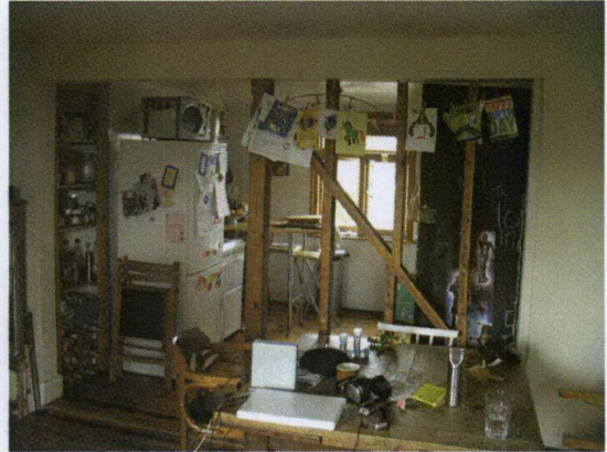
REAR ROOM showing exposed studwork
