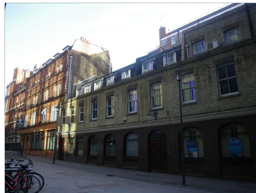
Figure 5.10: View of the buildings on the eastern side of Hand Court
