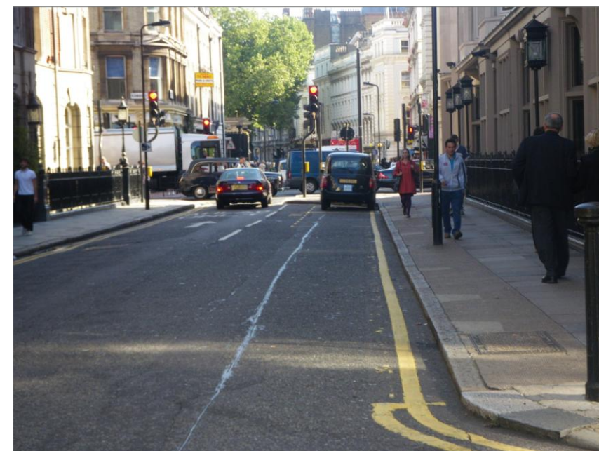
Figure 5.8: View of the site showing the single yellow line and taxi stand
