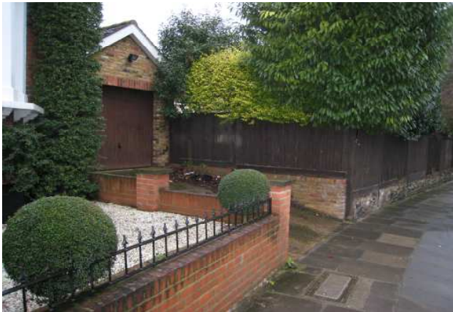
Boundary fence next to garage
