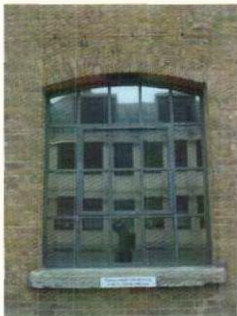
Figure 2 - Typical Windows at 19 Mandela Street
