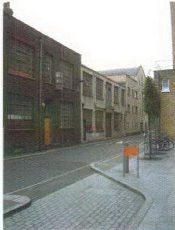
Front Elevation - View towards Plender Street
