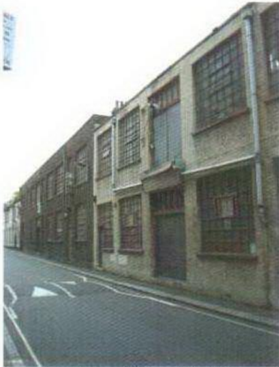
Front Elevation - View towards Pratt Street
