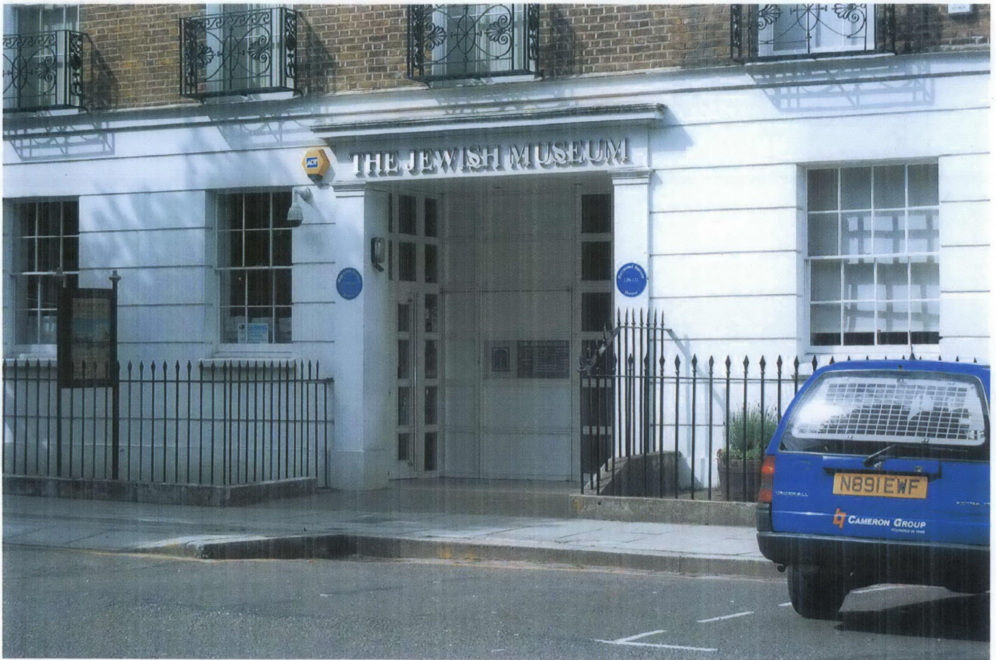
PHOTOGRAPH OF EXISTING CCTV CAMERA AND ALARM SOUNDER PHOTOGRAPH TAKEN PRIOR TO RENOVATIONS COVERED BY APPROVED APPLICATIONS 2006/5403/P AND 2006/5404/L
