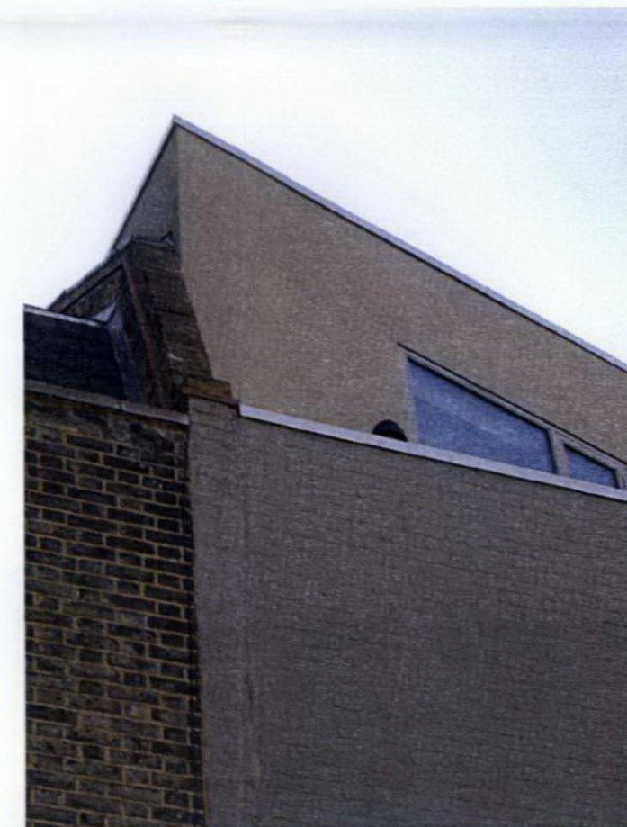
precedent for aluminium parapet coping
