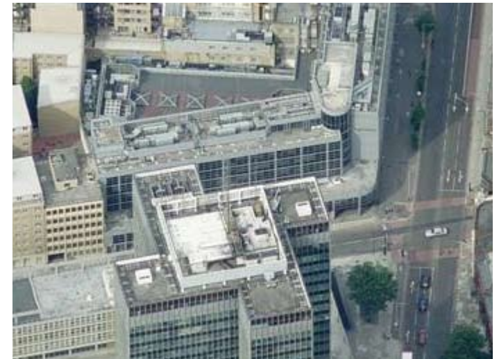
Figure 2 shows an aerial view of the site context.
