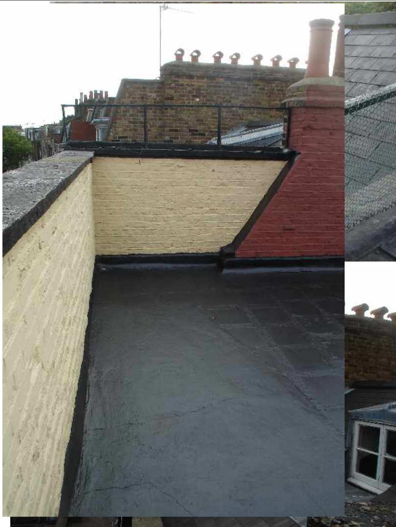
Rear Part of Roof Terrace looking towards 74 Delancey St
