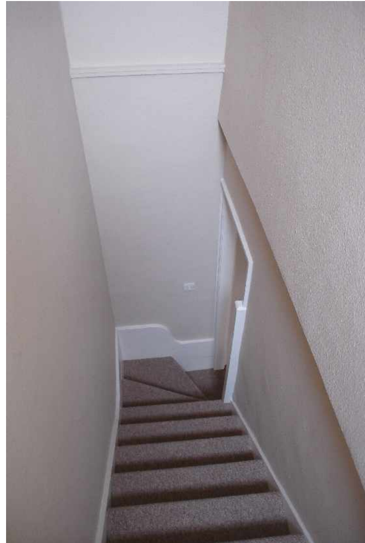
2 nd Floor Stair rising to Roof Terrace
