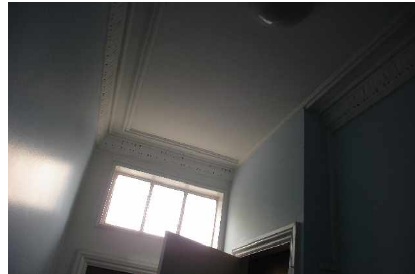
Ground Entrance Lobby – Existing Cornices
