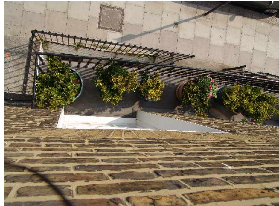
Front Elevation and balcony of 76 Delancey St (from 2 nd Floor)
