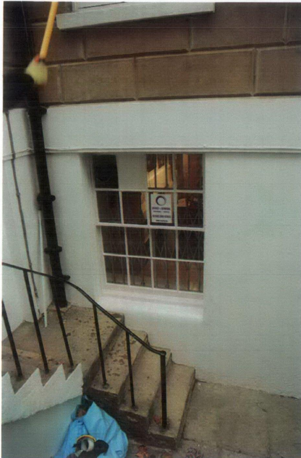
Photo 4 - Existing window W11
