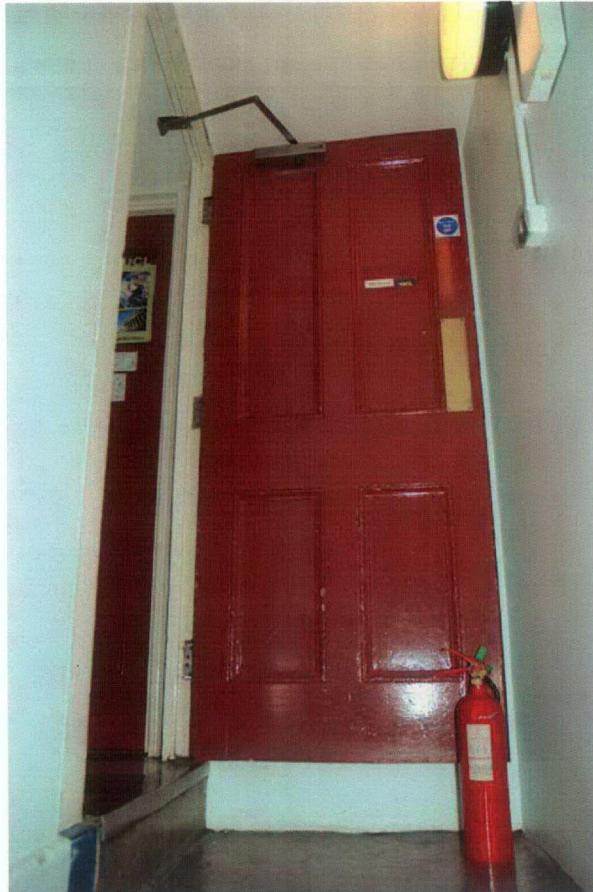
Photo 3 - Existing door DG4.2
