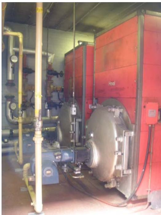
Image 4 – Boiler House Interior
