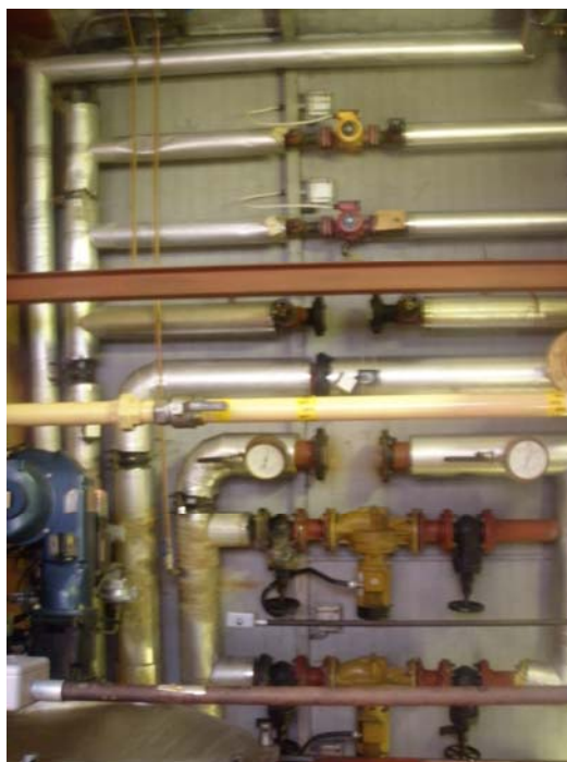
Image 5 – Boiler House Interior
