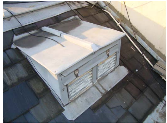
Rear Roof Ventilator
