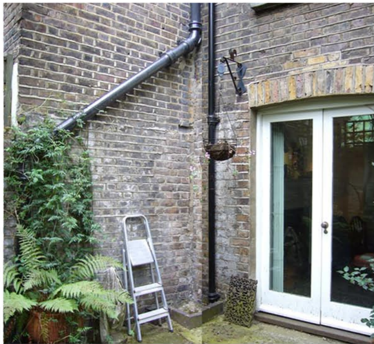
Lower ground floor patio
