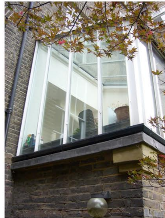
Ground floor conservatory
