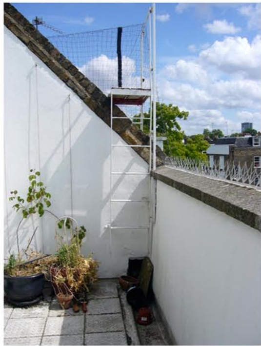
Top floor front terrace
