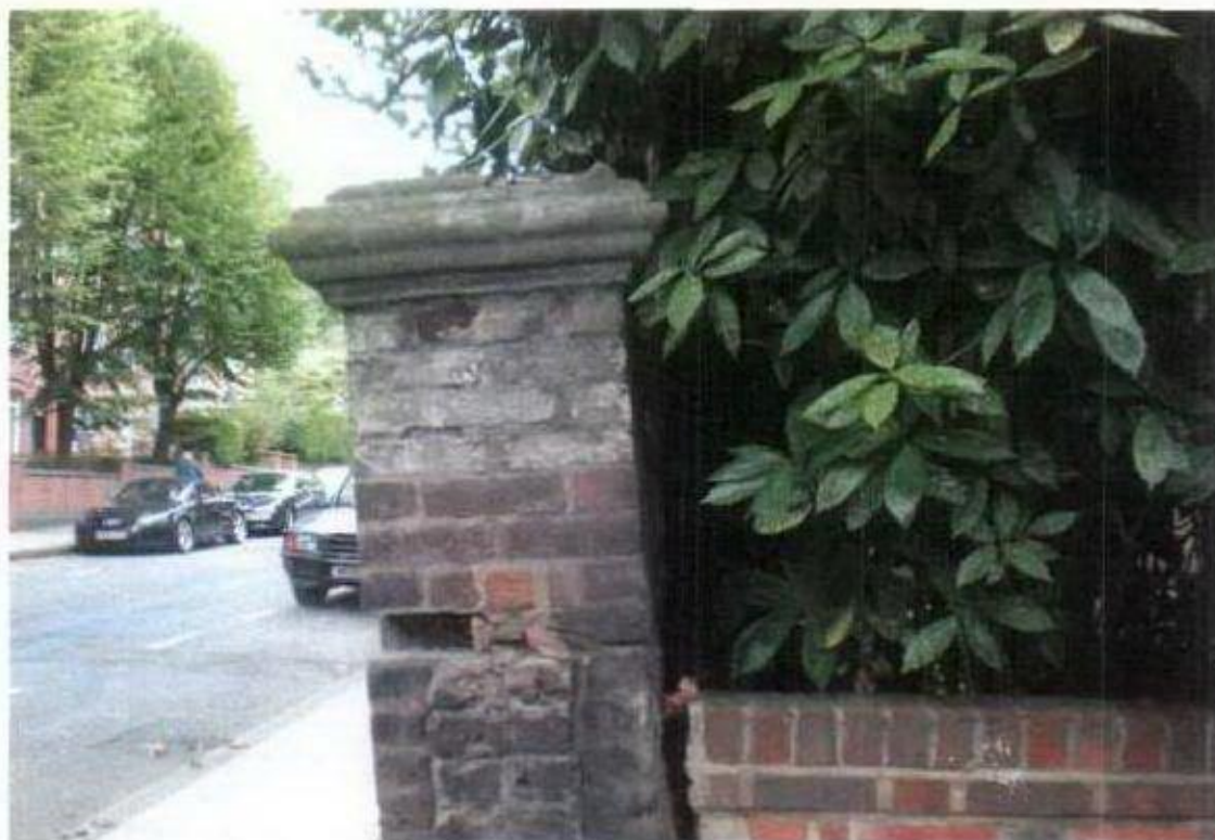
TOP SECTION OF PIER TO BE DEMOLISHED
