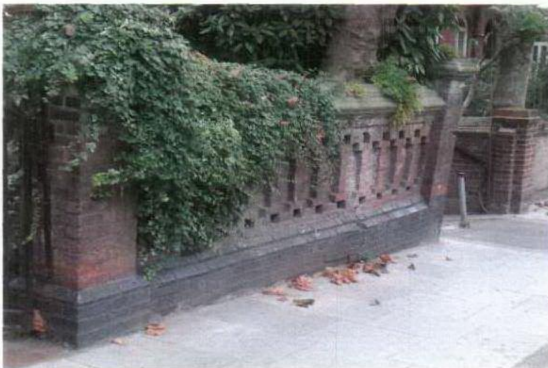
'LEAN' AND CRACKING TO SECTION OF WALL TO BE DEMOLISHED
