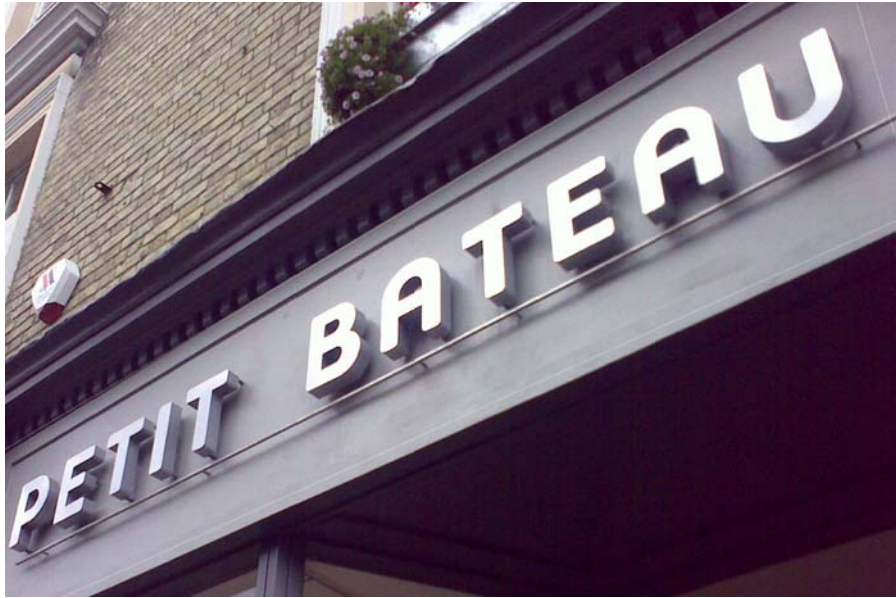
TYPICAL DETAIL OF REAR-ILLUMINATED S/S LETTERING
