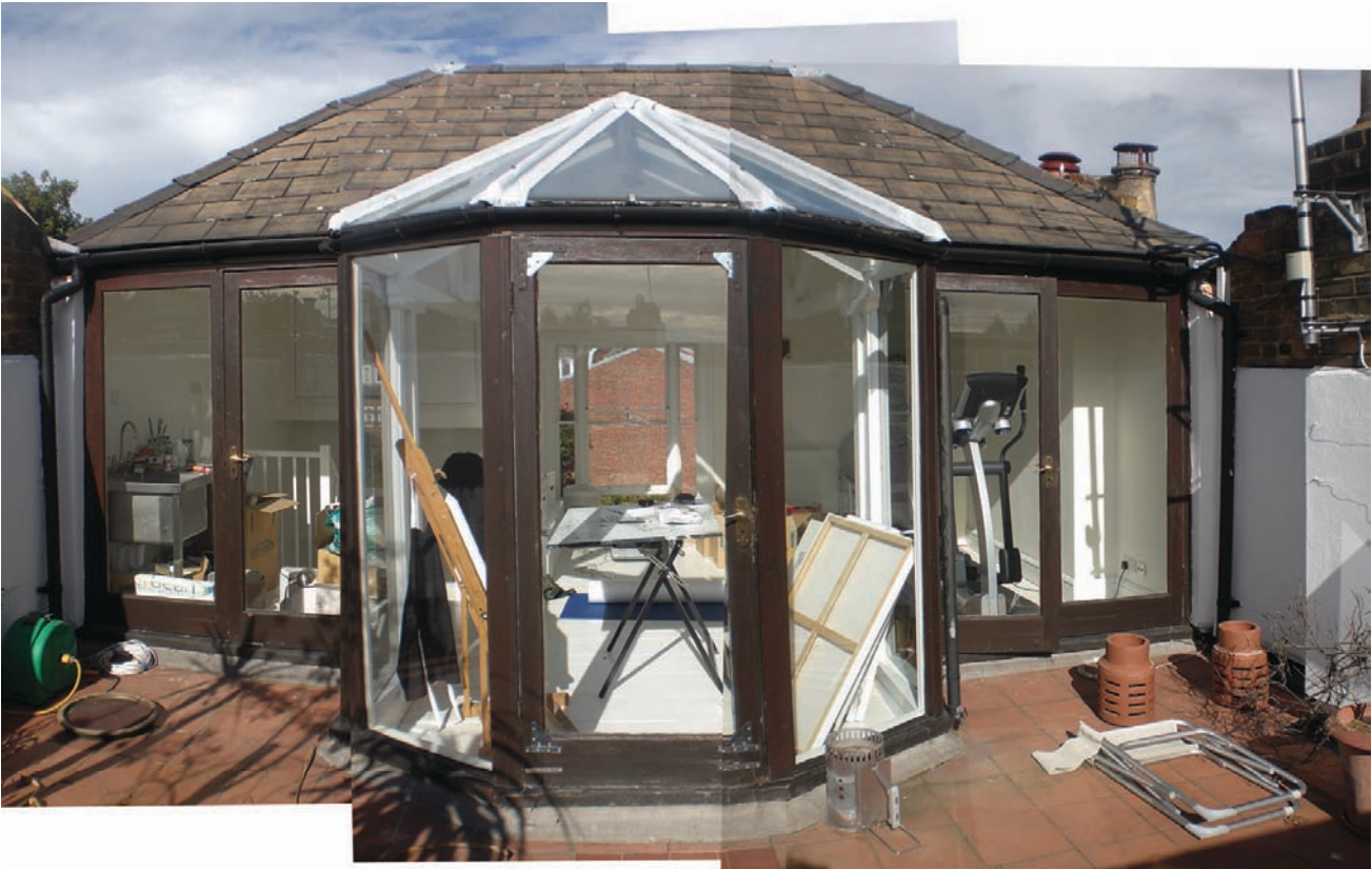
SITE PHOTOGRAPH SHOWING EXISTING ROOFTOP STUDIO ROOM
