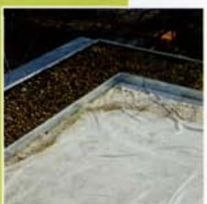
■ Where the roof does not have a perimeter parapet wall, the RDT Edge Profile provides one possible solution to the problem of how to retain the garden elements, whilst still allowing the free flow of
