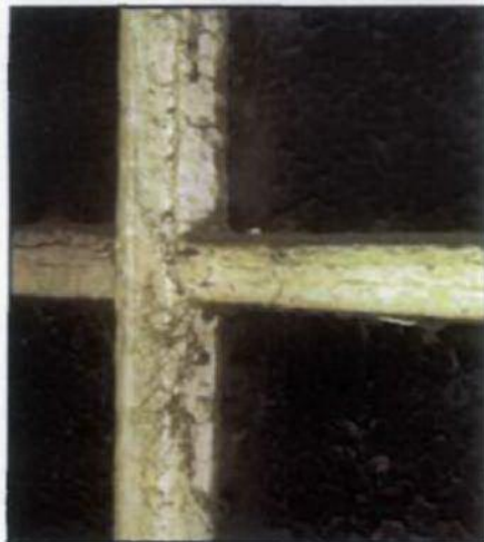
3) Existing Metal Horizontal Glazing Bar Detail
