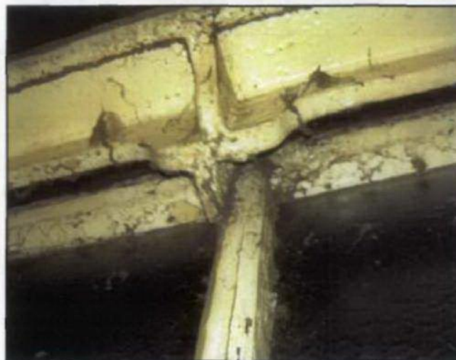
4) Existing Timber Glazing Bar Detail - Horizontal & Vertical Bars Similar
