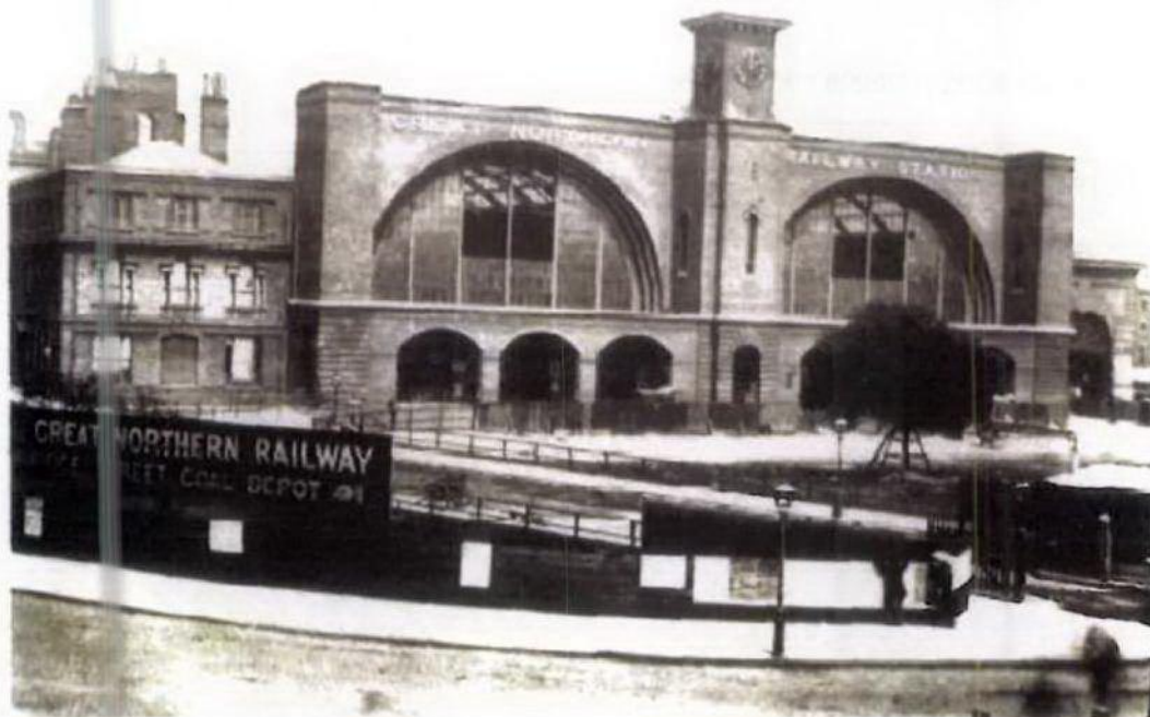
2. Photograph showing glass removed from centre sections
