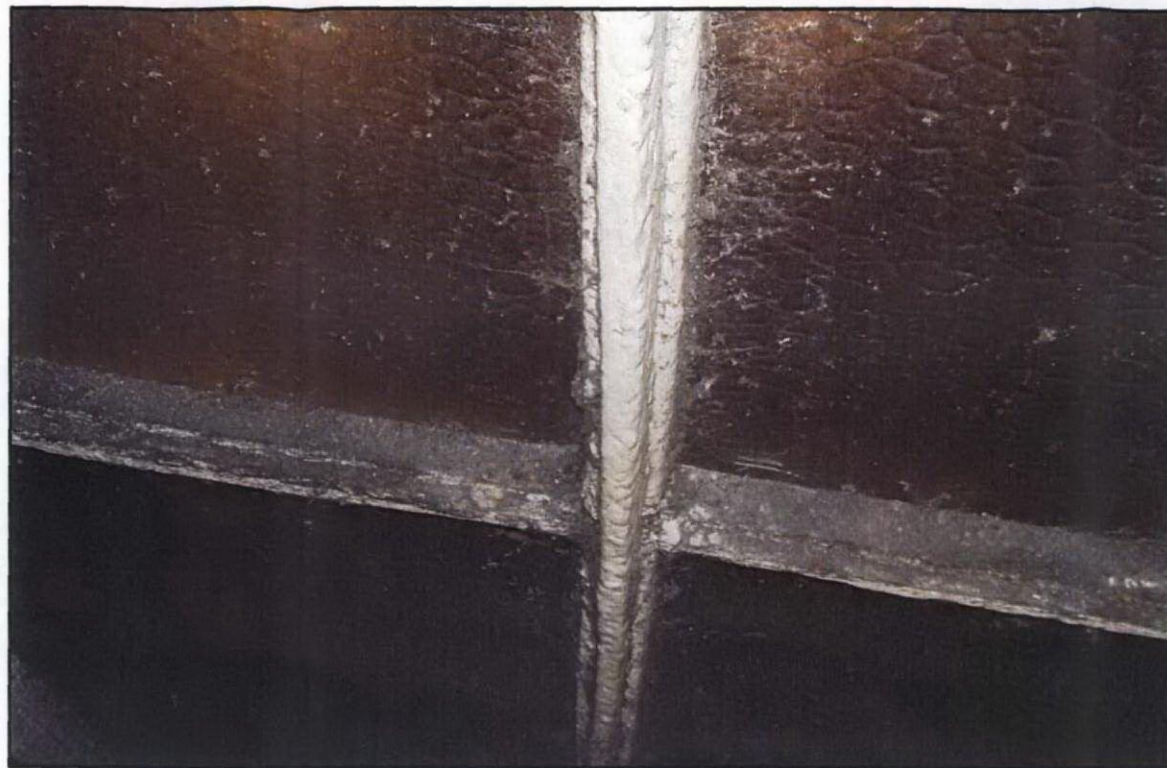
2) Existing Metal Vertical Glazing Bar Detail
