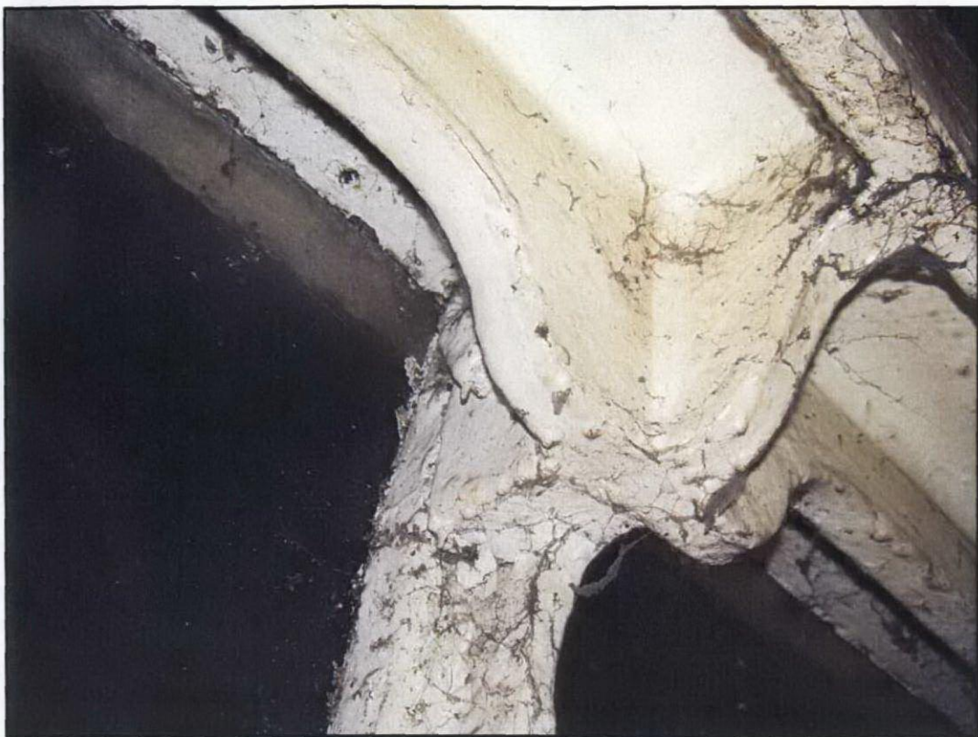
1) Existing Metal Vertical Glazing Bar Detail
