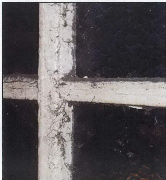
3) Existing Metal Horizontal Glazing Bar Detail
