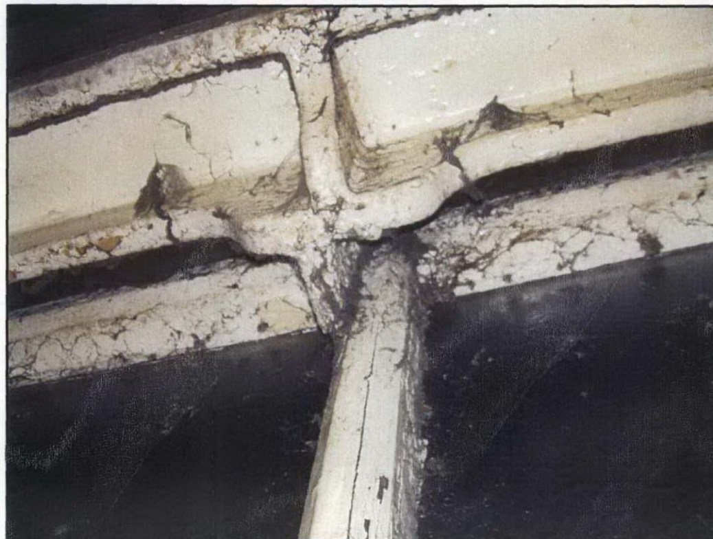
4) Existing Timber Glazing Bar Detail - Horizontal & Vertical Bars Similar
