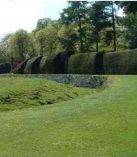
boundary type 4: haha (edge palisade retaining wall becomes barrier)
