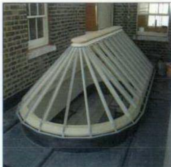
Replacement skylight in the roof of No. 14
