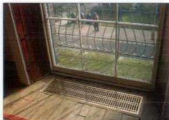
in No. 14 - radiators were recessed into the floor
