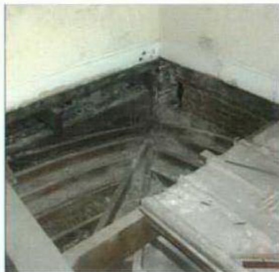
Soane's complex floor structure on the second floor of No. 14
