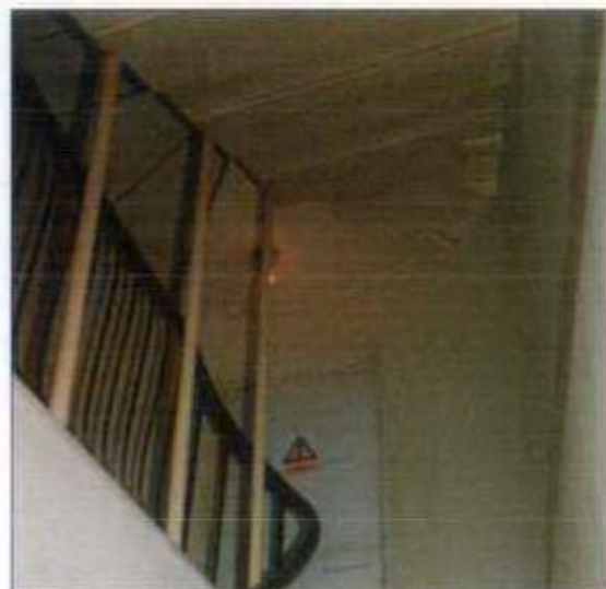
C20 propping to the No. 12 staircase which needs to be replaced
