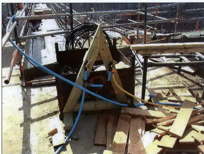
An example of a temporary watering system rigged up on site to provide an adequate mains watering feed to different roof areas.
