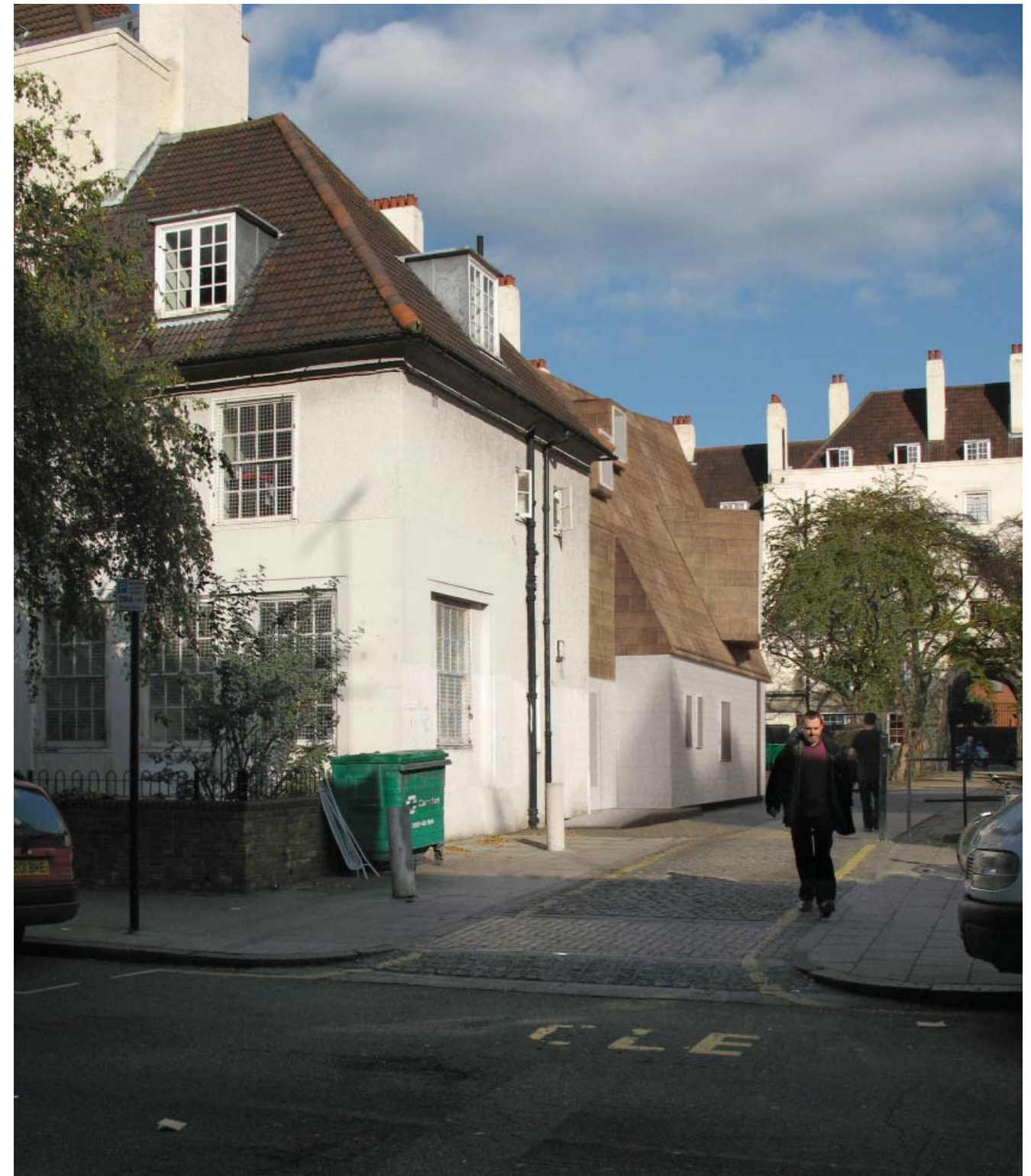
2. View from Chalton Street into the northern courtyard The new side entrance marks the transition between the existing building and the new extension. The variety of windows in different sizes echo the situation in the adjacent elevation of the south tower.
