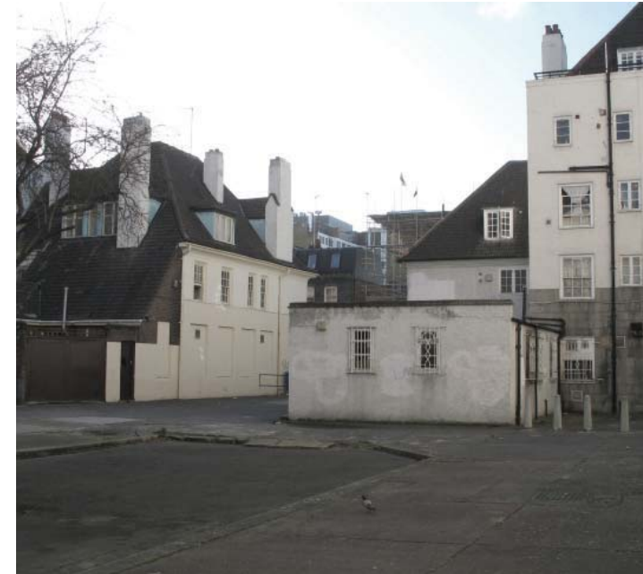
Photograph of existing single storey extension
