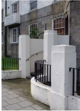
Piers flanking entrances
