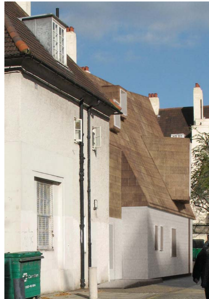
The metal shingle system allows for clean detailing, maintaining the buildings formal identity
