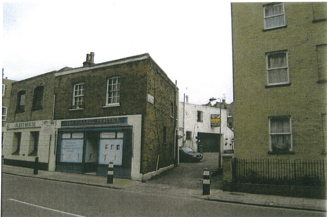
2. APPROACH FROM HIGHGATE ROAD
