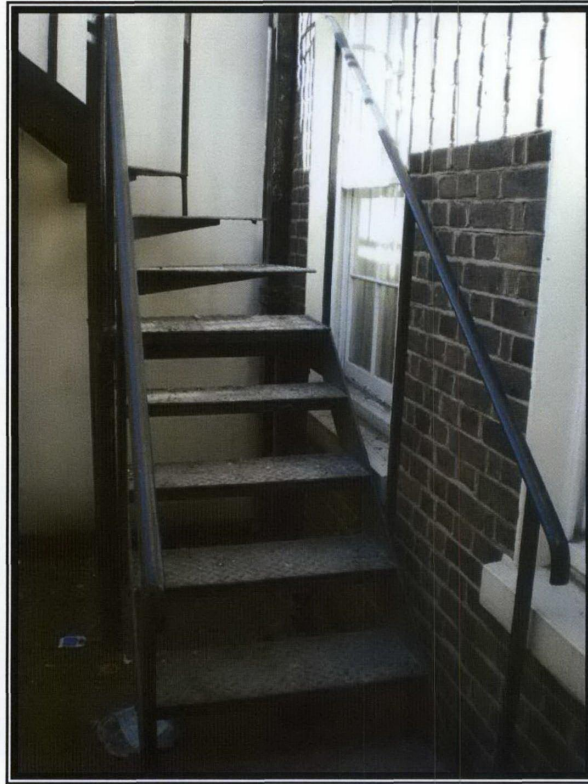
Photograph 265 – Metal stairs down to light well
