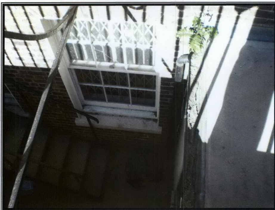
Photograph 264 – Front light well
