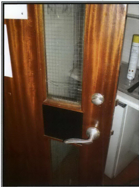
Photograph 211 – Glazed panel cracked within door
