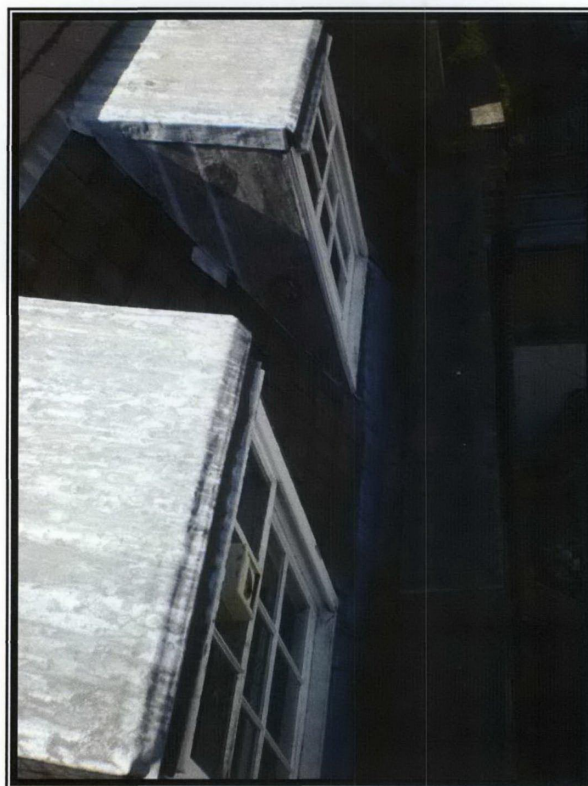
Photograph 223 – Lead covered dormer windows
