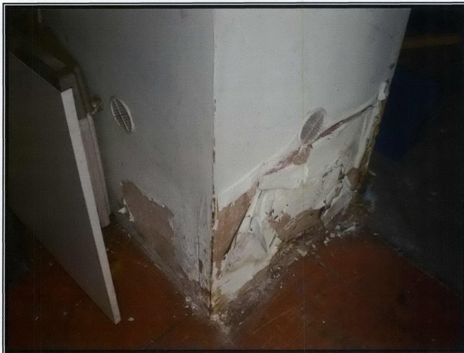
Photograph 210 – Damp damage to base of column
