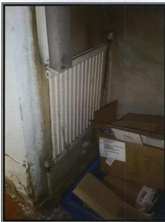
Photograph 214 – Damp damage to wall and damaged light fitting and radiator pipework
