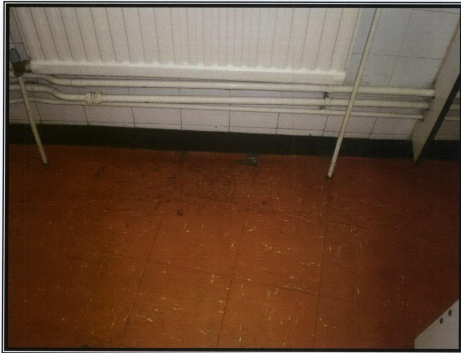
Photograph 185 – Damage to floor finish
