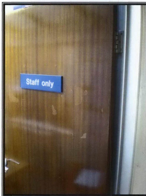
Photograph 178 – Door coating chipped and worn
