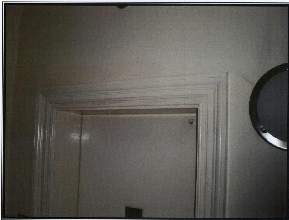
Photograph 190 – Horizontal crack above lift door opening
