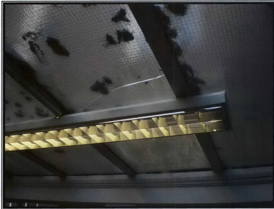
Photograph 173 – Crack in glazed roof pane
