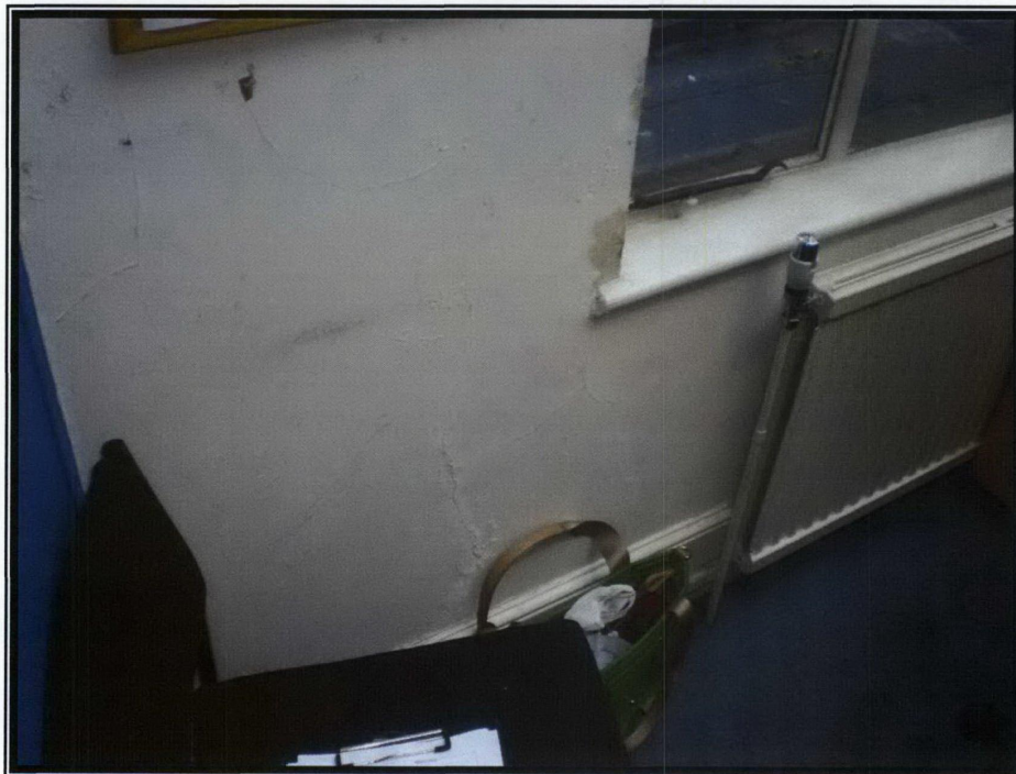
Photograph 176 – Cracked and damp plasterwork to western wall
