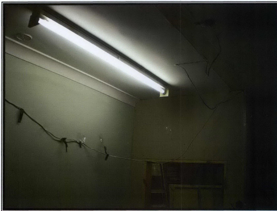
Photograph 198 – Ceiling damaged and wiring loose where partition wall removed
