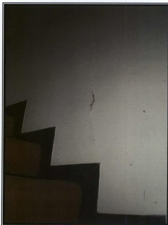
Photograph 188 – Plasterwork cracked above stairs
