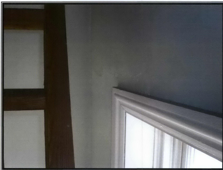
Photograph 50 – Blown plasterwork and crack running to left of window opening
