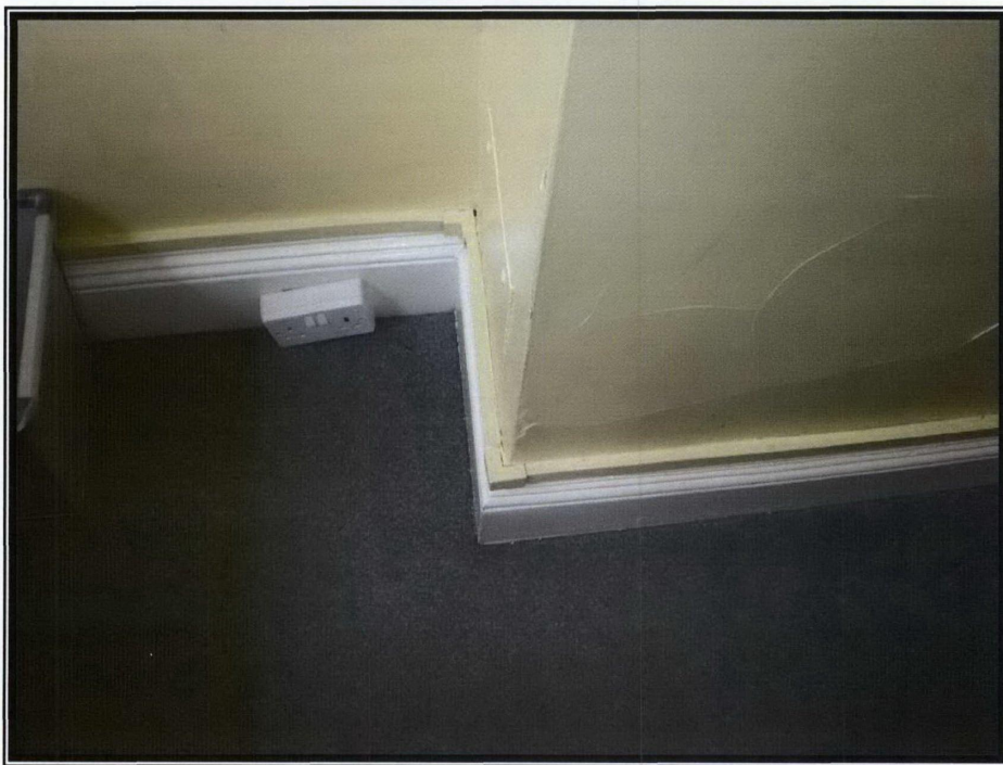
Photograph 62 – Displaced double socket to left of chimney breast
