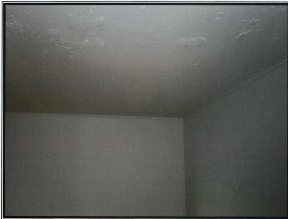
Photograph 52 – Separation between exposed ceiling partition walls
