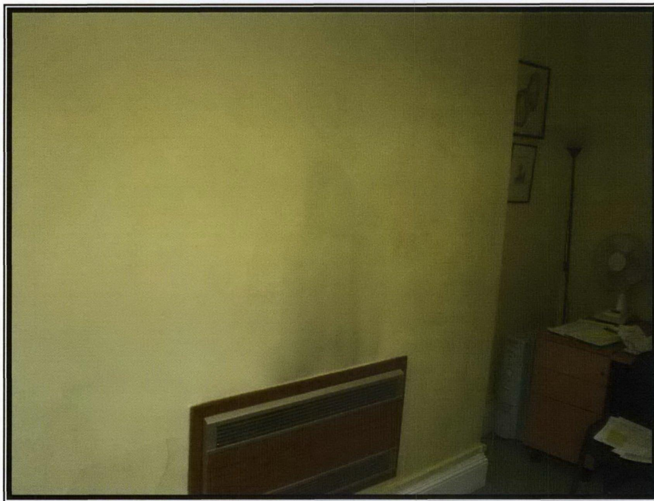
Photograph 61 – Blown plasterwork to chimney breast
