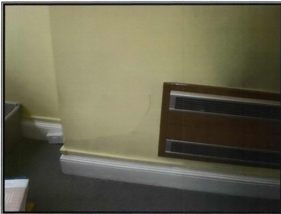
Photograph 60 – Blown plasterwork to chimney breast
