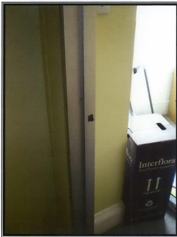
Photograph 56 – Door latch-keep damaged
