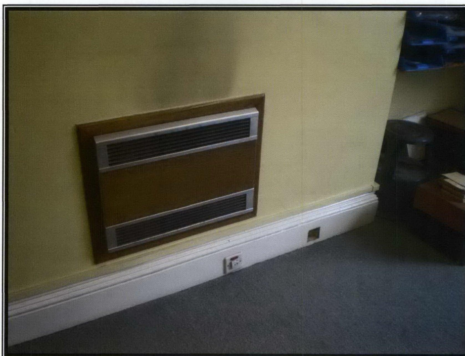
Photograph 74 – Cracked plaster to left of heater and missing socket in skirting
