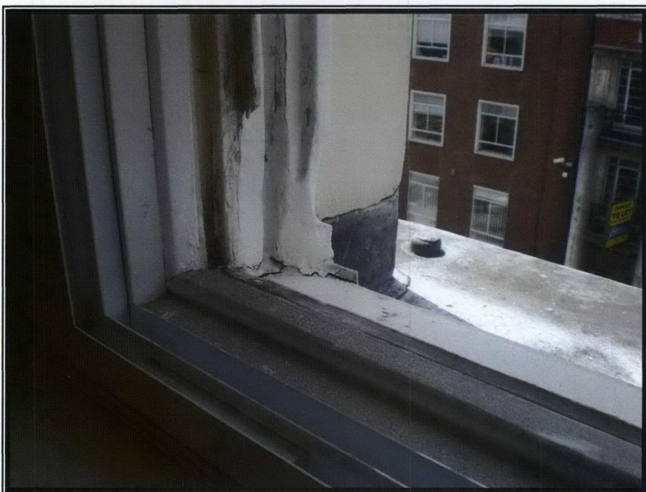
Photograph 12 – Sash frame damaged and filled
