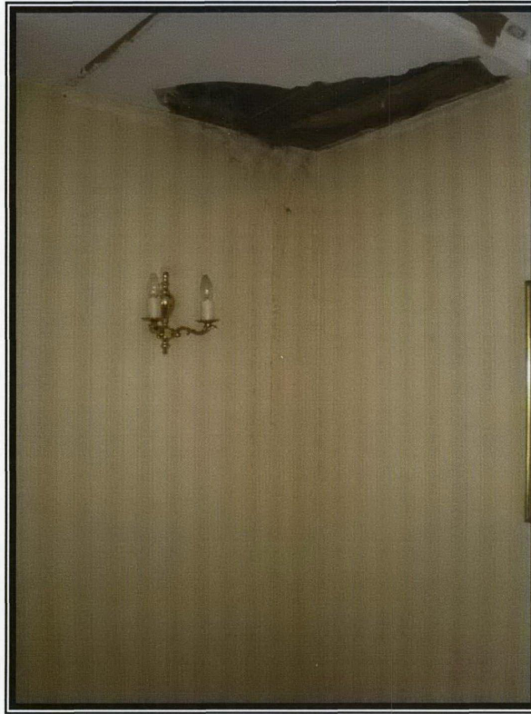
Photograph 3 – Damp staining to wall and damaged wall paper coverings
