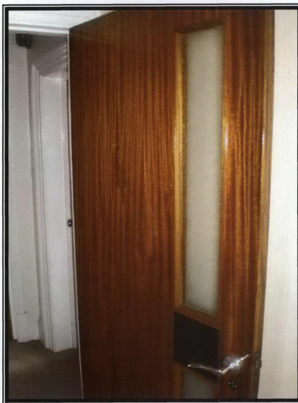
Photograph 17 – Chipped varnish to door
