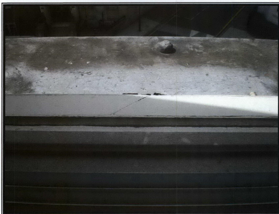
Photograph 13 – Scarfed joint repair to timber sill
