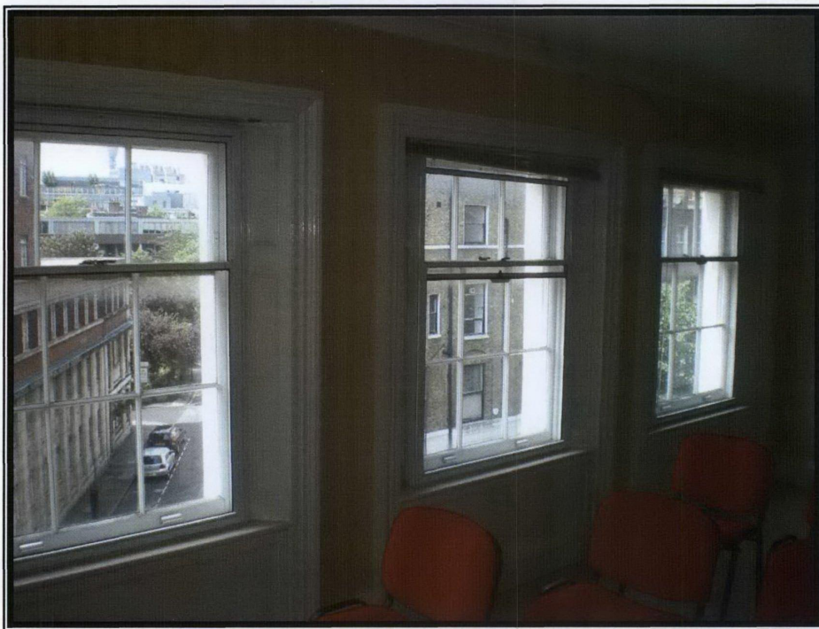
Photograph 11 – Secondary glazing to window openings
