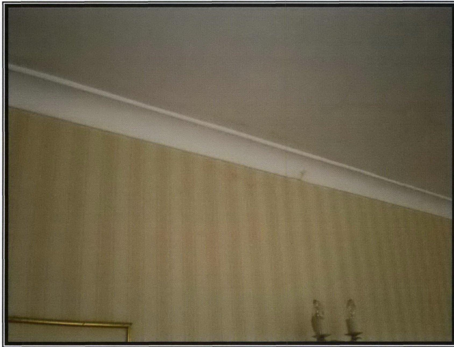
Photograph 5 – Water staining to ceiling and coving along eastern wall
