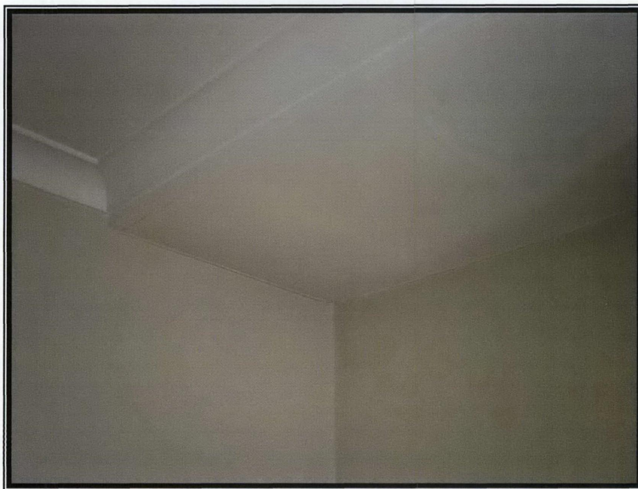
Photograph 18 – Cracking to ceiling soffit and coving within north western corner
