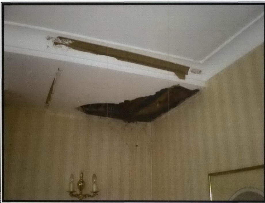
Photograph 2 – Displaced plaster board ceiling and exposed water damaged roof structure
