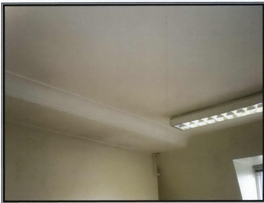
Photograph 19 – Separation to plaster board joints
