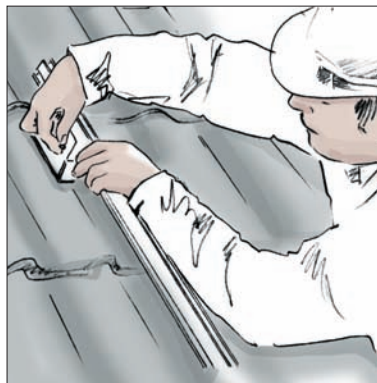
6. Attach rails to brackets. 7186230
