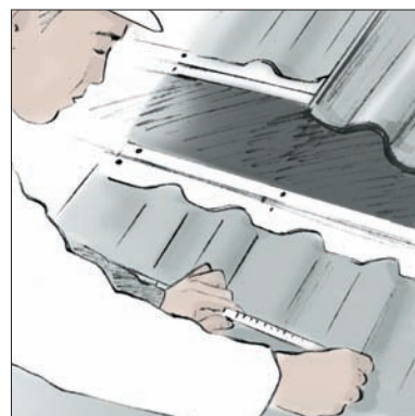
2. Measure roof & remove tiles.
