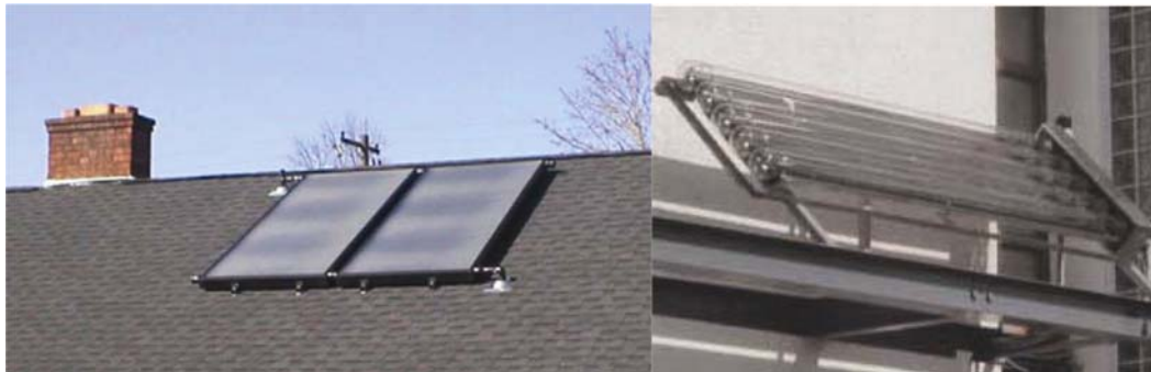
Figure 2: Roof mounted solar thermal systems; flat plate (left), evacuated tube (right)
