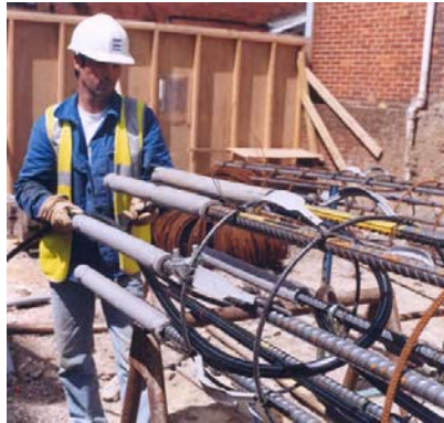
Figure 4: The preparation of GSHP heat exchanger loop in 'Energy Piles'
