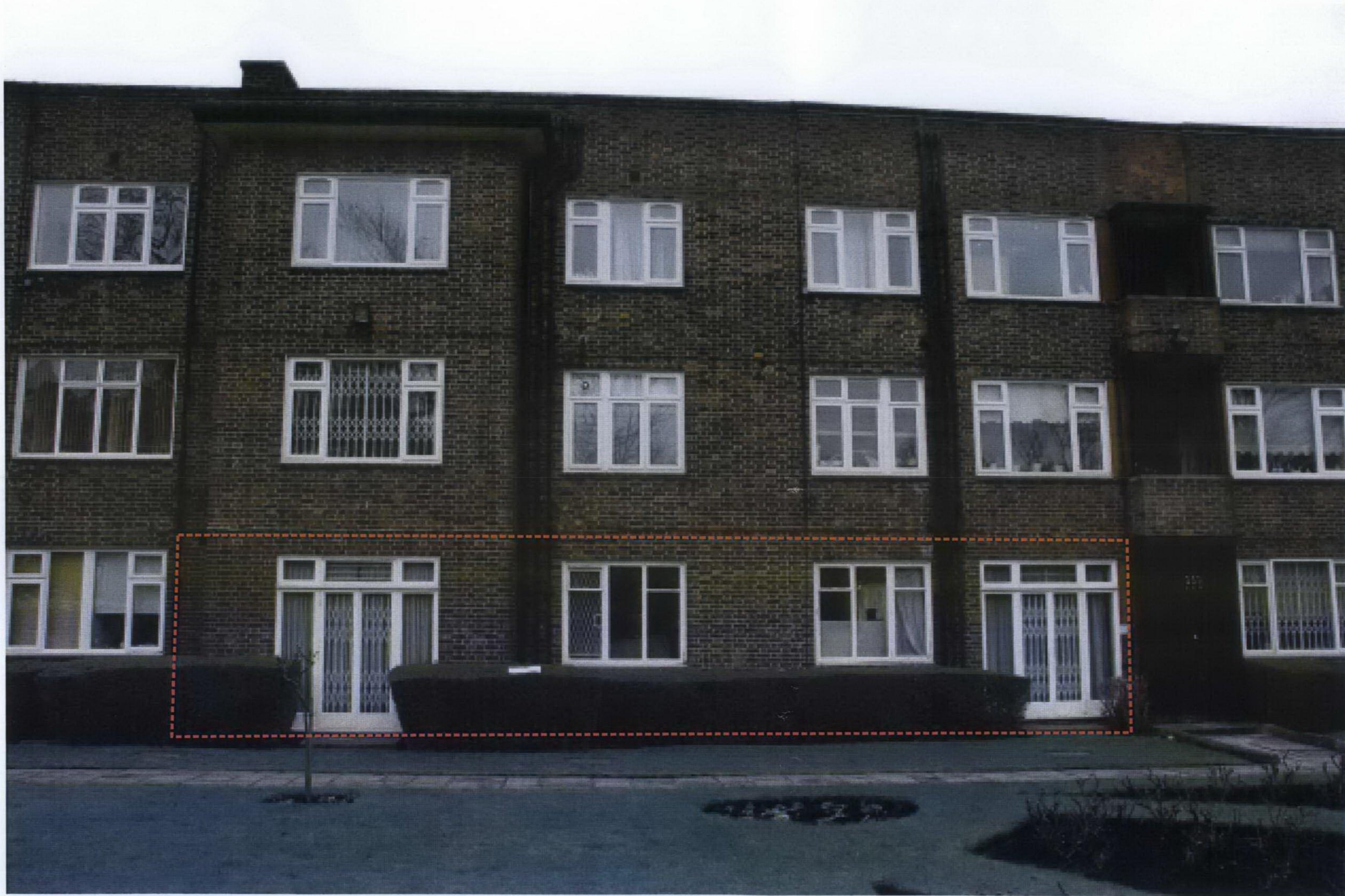
Image 5- existing garden elevation with Steel framed window and doors
