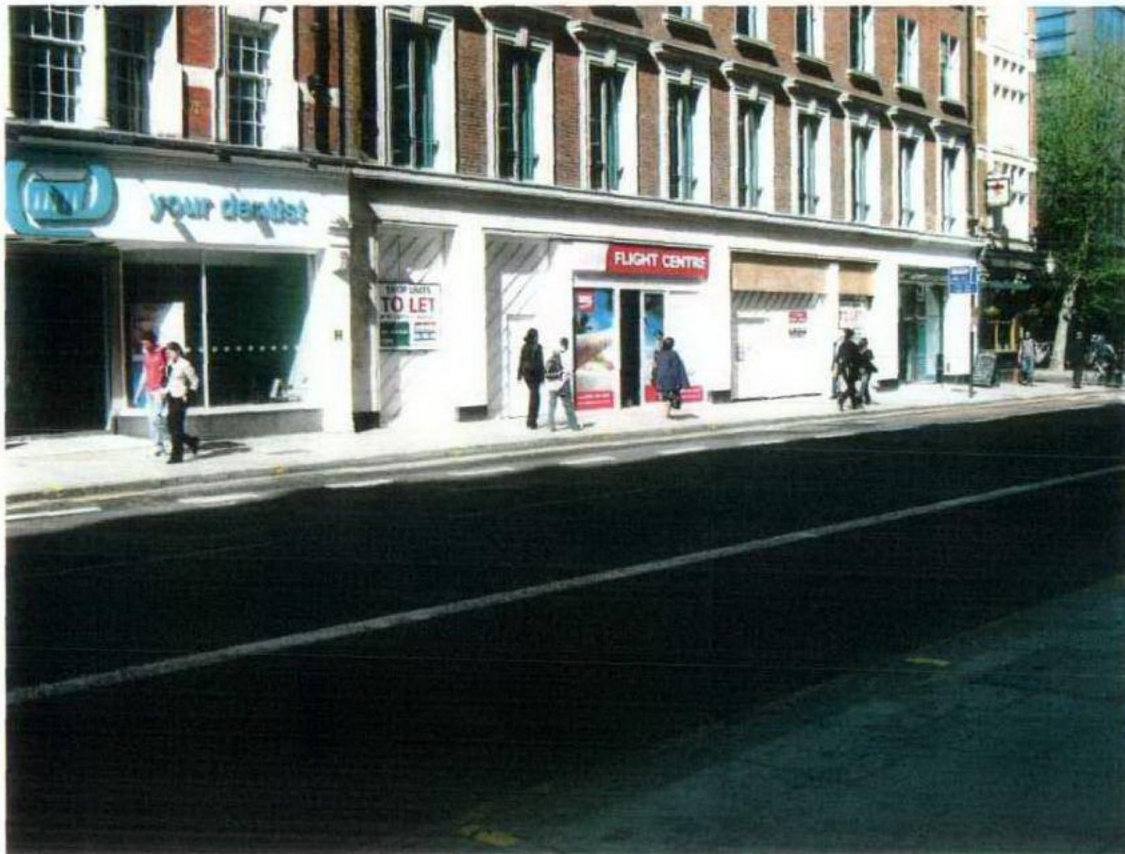
EXISTING FACADE UNIT 1. 75 High Holborn. LONDON WC1V 6LS
