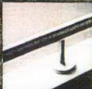
SS, 1F Satin Polished Stainless Steel wallup handrail connected at maximum 1200mm centres to Stainless Steel stem brackets with concealed flange.
