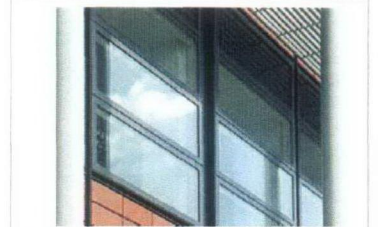
2 Vallat 200 Thermally broken aluminium sections RAL 9005 RAL Cyprium
