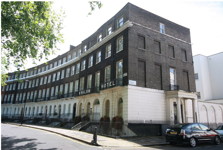
View of the building as seen from Cartwright Gardens
