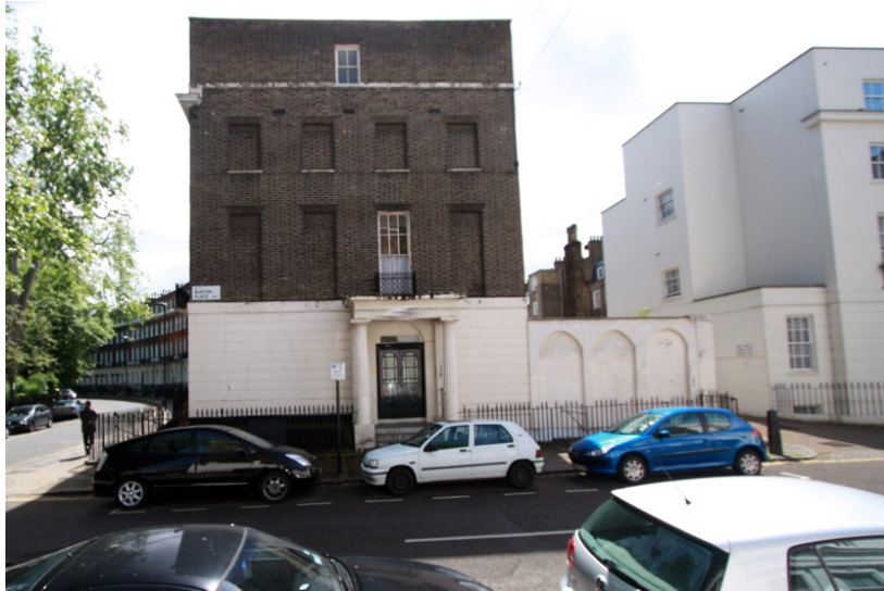
View of end elevation as seen from Burton Place
