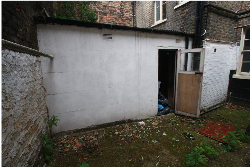
Proposed location for air conditioning condensers, lower ground.
