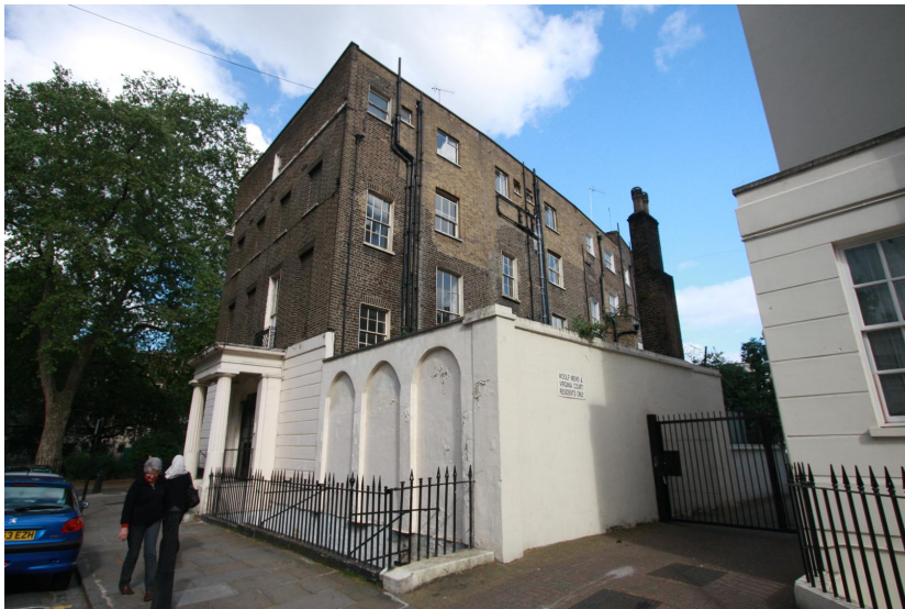
Rear wall behind which ground floor bedroom G07 will be housed
