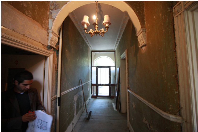
Existing features within reception lobby at ground floor
