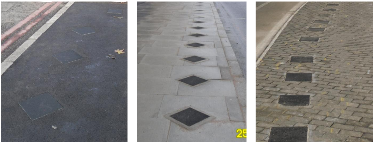
Figure 4: Examples showing finish achievable with the foundation square box cover
