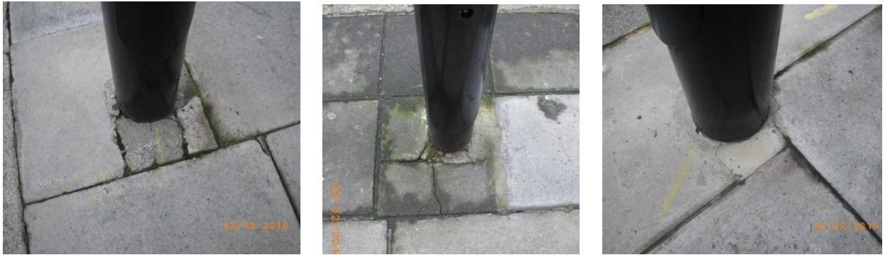
Figure 5: Examples of paving finishes around curved street furniture
