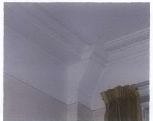
Image 2: Non original ductwork to be removed
