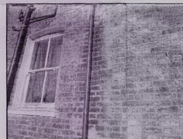
rear elevation brickworks
