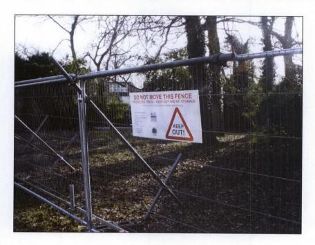
Wooden Framework with 'Heras' type panels attached.
