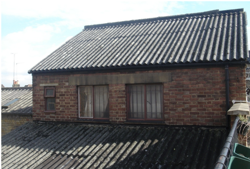
Photo 2: West elevation of existing building from terrace to 132 Fortress Road.
