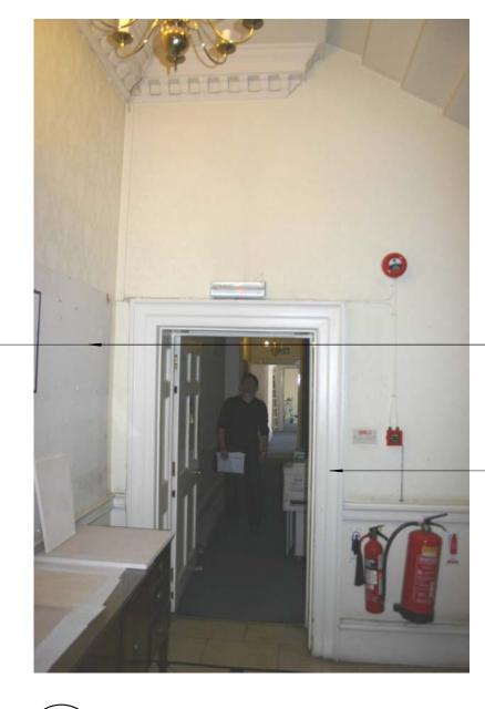
Proposed location of possible new opening in masonry wall linking No's. 7 and 8 Southampton Place. New door to match existing door DG04. See door details - drawing No. 0264
