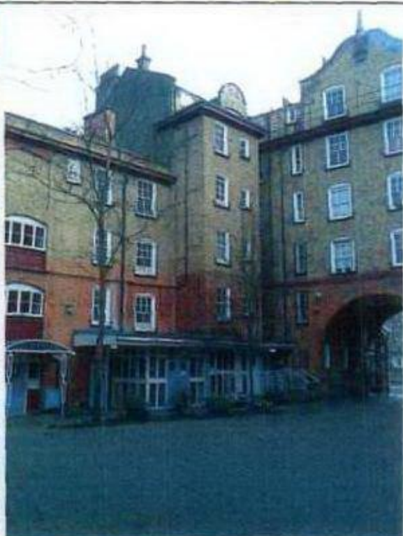
View of T2 and T1 looking south east
