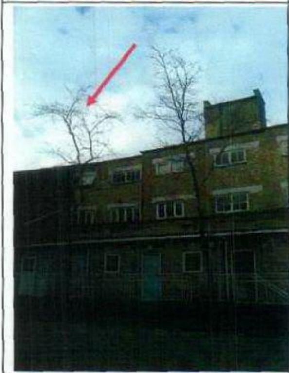
T4 and T5 looking north
