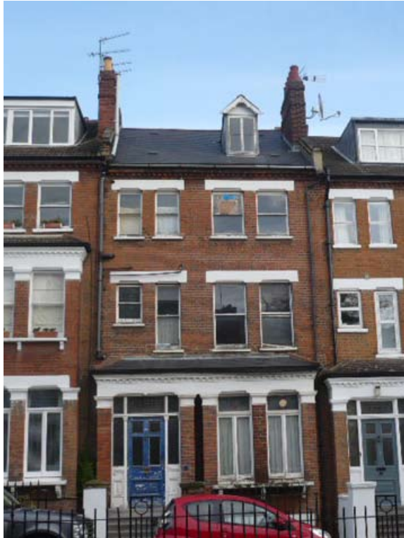
Existing Elevation of 44 Primrose Gardens with original dormer window
