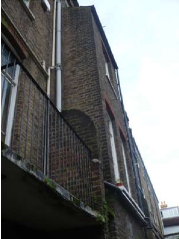
Detail photograph of rear of property and adjacent extension
