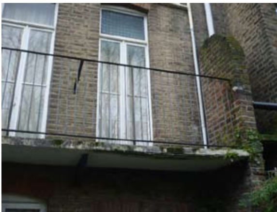
Detail photograph of rear of property.
