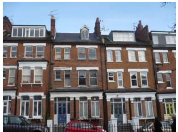
The enlarged dormer windows of adjacent properties
